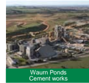
Waurn Ponds Cement works
