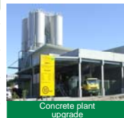
Concrete plant upgrade
